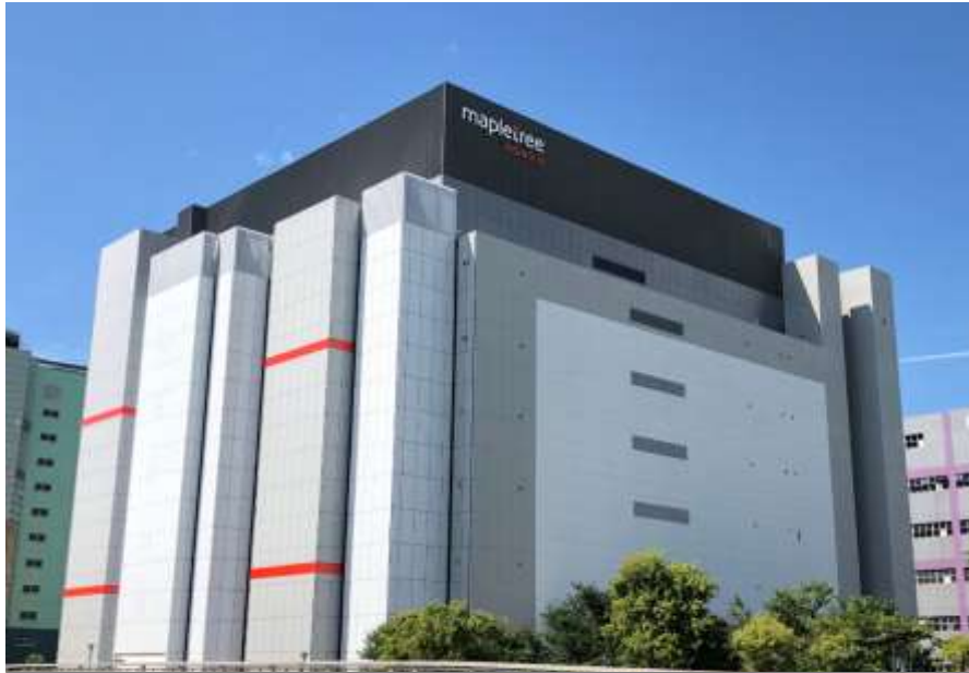
7 Tai Seng Drive (after upgrading into a data centre)
